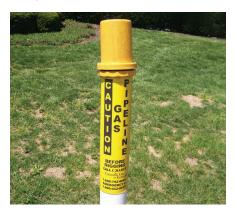
They are generally placed wherever needed to indicate the presence of a pipeline, such as where a pipeline easement intersects a street, railroad or river and in heavily congested areas. Line markers are not always directly over the main but indicate that a gas pipeline is in the area. The absence of above-ground markers DOES NOT indicate that there are no gas lines in the area.
